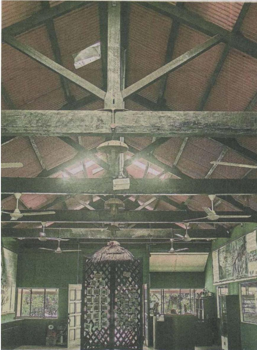
The ceiling beams have visible rough marks possibly indicating they were cut using a push-pull long handsaw commonly used over a century ago.
